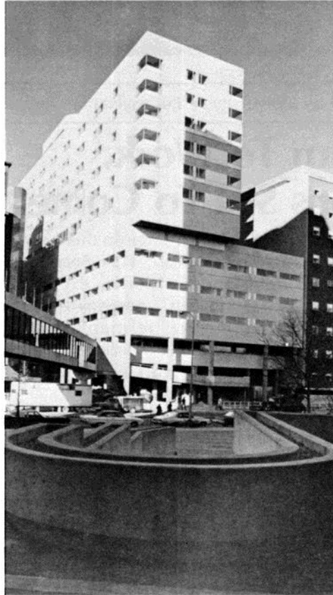
The new Silverstein Pavilion, seen here from the Hilton Hotel, is rapidly nearing completion, aided by a number of Operational Services departments.
